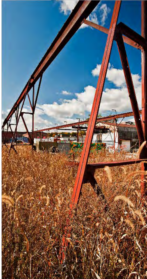
Agricultural - Pivot irrigation/Feedlot catwalks.
